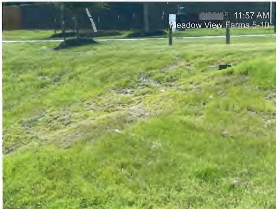
Drain line with erosion
