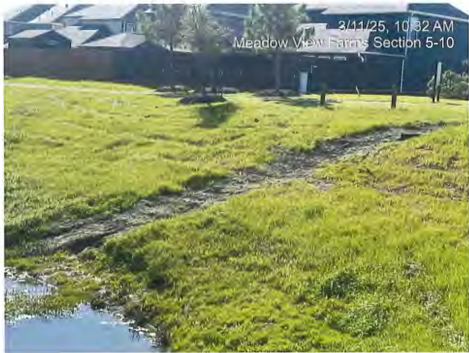
Drain line with erosion
