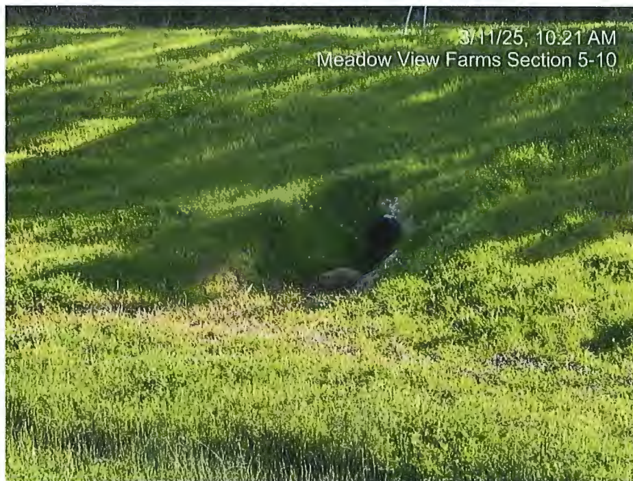
Drainage pipe doesn't extend to the toe of the pond, East side of pond
