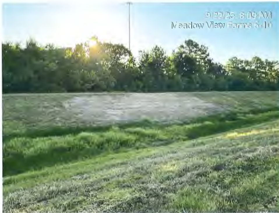
Filled in the washed-out area near the Northeast corner of the pond
