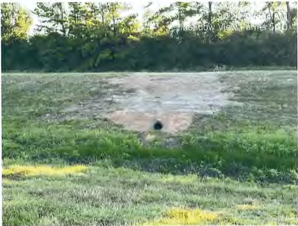
Drainage pipe extend to the toe of the pond, East side of pond
