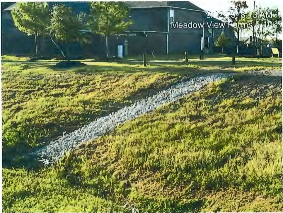
Drain line with riprap
