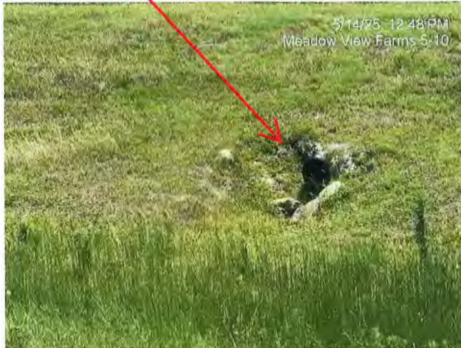
Drainage pipe doesn't extend to the toe of the pond, East side of pond
